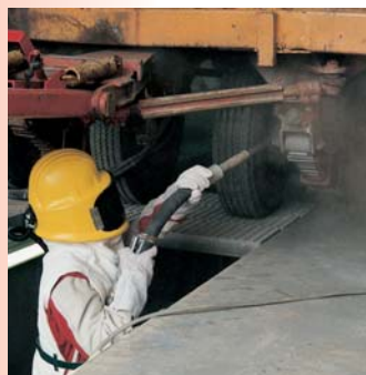
LKW-Strahlen Truck sandblasting
